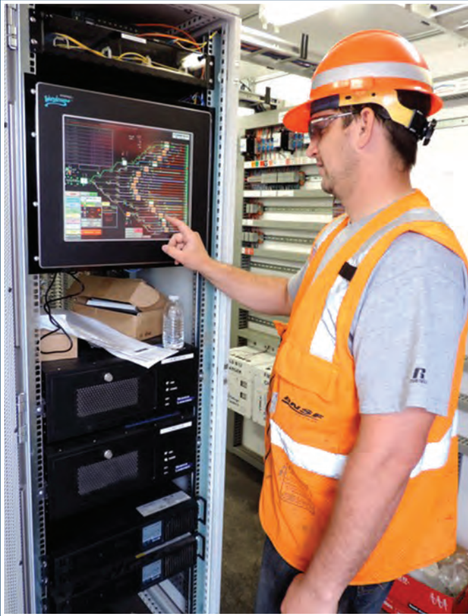
Jace Spurling, Local 119 member and Signal Electronic Technician, BNSF Lincoln Terminal, is shown above programming a hump yard retarder computer.
