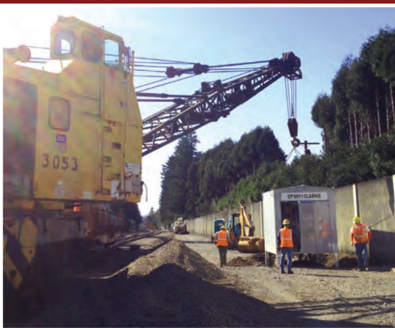
Signalmen Ian Johnson and Joe Colotti, both members of Local 111, set a 8x10 CP house with help from Maintenance of Way workers Scott Braddock (Crane Operator) and Greg Lee (Equipment Operator).
