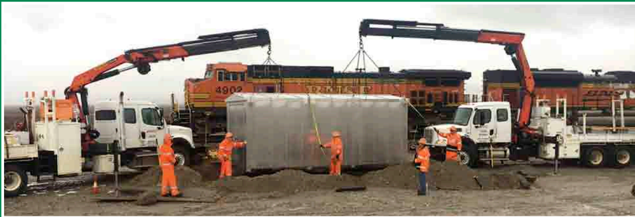
Spokane signal crew setting a 10'x22' Bungalow for the new East Needles control point on the BNSF CA Division. Pictured from left to right: Wayne Newby, Ray Opfer, Steven Ayers, Carlos Soliz, and Pete Overbee, all members of Local 188.
