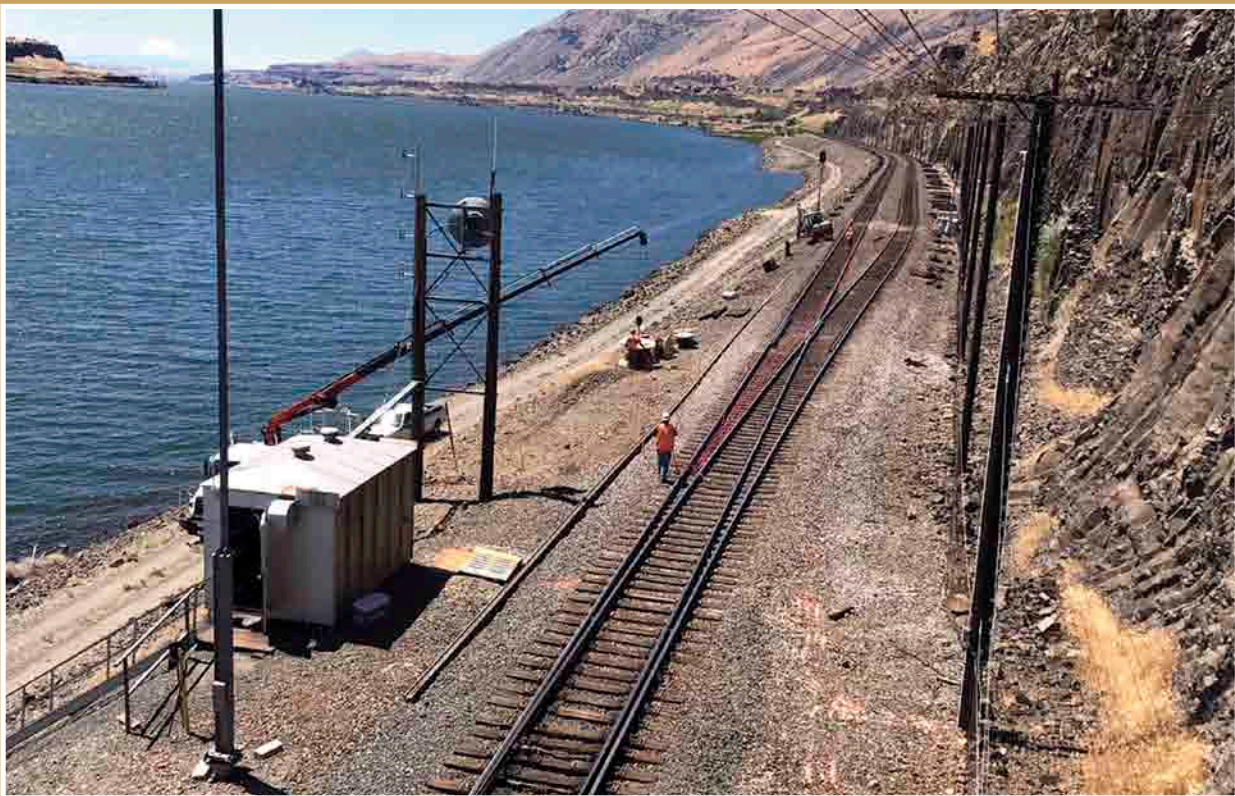
Tacoma Mobile Signal crew installing a new signal house, new cable, signal and switch, and updating slide fence circuits along the Columbia River, near Mt. Hood at the East Towal, Northwest Division, Fallbridge Sub Division. Pictured are Local 188 Members James Halbert, Brad Webb, Nick Aldridge, Steve Griffis, James Kyriss, Adam Minsker, John Carwile, Colby Holt, and Keith Dybdahl.
