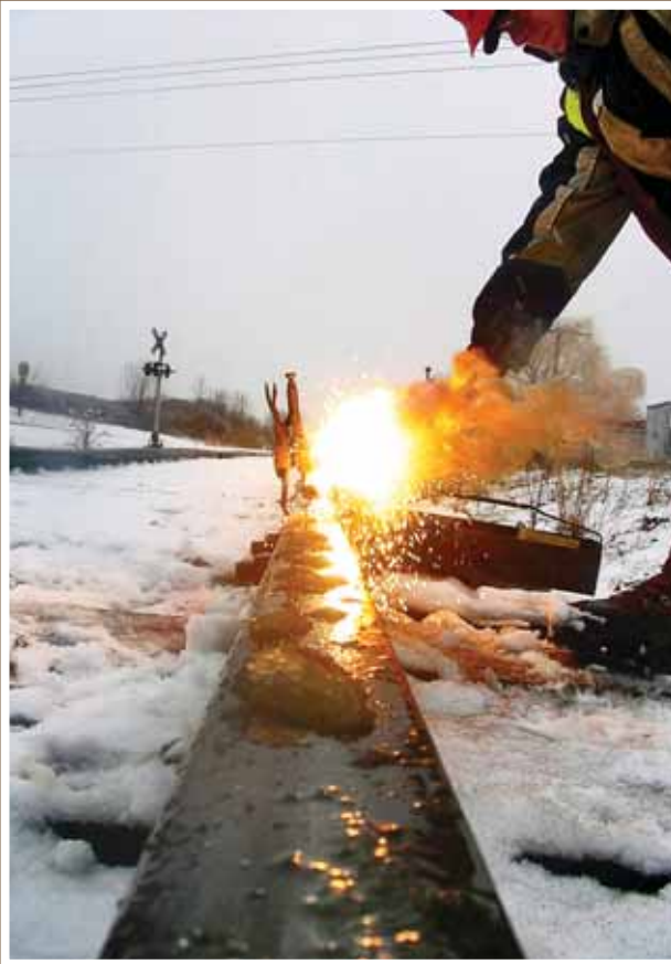
Rail bonding after a recent wet snowfall on the Wisconsin and Southern, Milwaukee Subdivision in Richfield, WI. Chris Roland quickly moves away from the spark applied to the bonding powders of a rail bond. Photo submitted by Chris Roland, Recording-Financial Secretary and member of Local 236.
