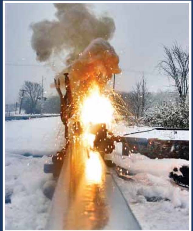
Rail bonding after a recent wet snowfall on the Wisconsin and Southern Milwaukee Subdivision in Richfield, Wisconsin. Photo submitted by Chris Roland, Recording-Financial Secretary and member of Local 236.
