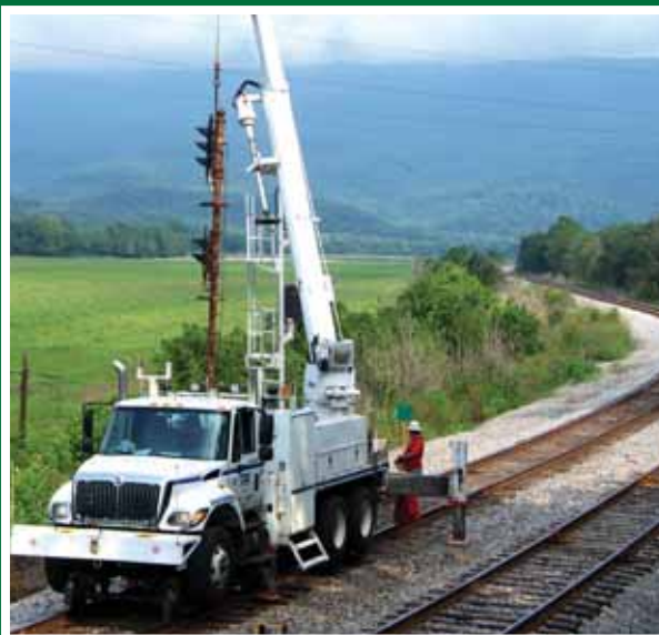
Scott Menix and Tim Cox, both members of Local 136, remove old signals during a cut-in at E.E. Haden. Photo submitted by Local 136 member C.A. Hawkins.
