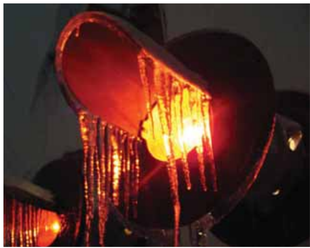
One of the worst ice storms in Kentucky history hit on January 27, 2009, crippling 101 counties and 75 cities statewide. The railroad was also severely impacted due to ice covered trees falling on approximately 100 miles of pole-line which is used to assist with the governing of train movement by providing adequate signals. Photo submitted by member D.J. Bocook — Local 176.
