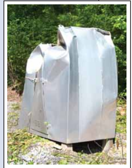
The photos above show a small aluminum signal shed near Robson, West Virginia, that was crushed by a falling oak tree. Photo submitted by Local 77 member and Local Chairman L.B. "Brad" Elliott.
