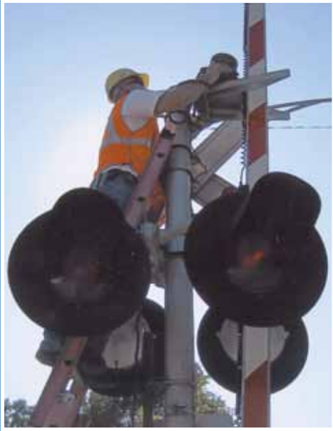
Photo of Signal Maintainer James "Jimmy" Hansen replacing a bell at the 103rd Street Crossing on Metra's Rock Island Division, Beverly Branch.
