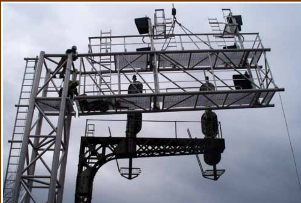
Matt Antes and Zeke Downey install a new cantilever arm on the Chesapeake and Ohio in Covington, VA.
