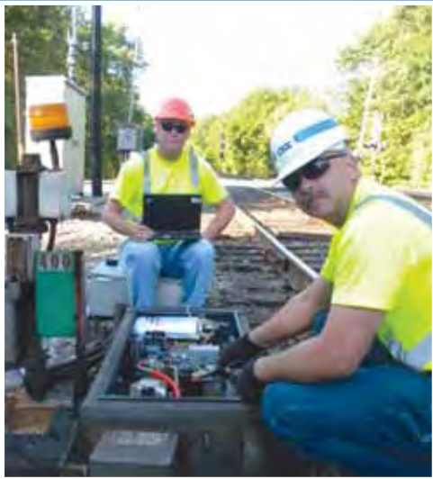
Lead Signal Maintainer Bill Cundiff, Jr. and Signal Maintainer Jason Wade, both members of Local 71, make adjustments to a radio-controlled switch in Evansville, Indiana.
