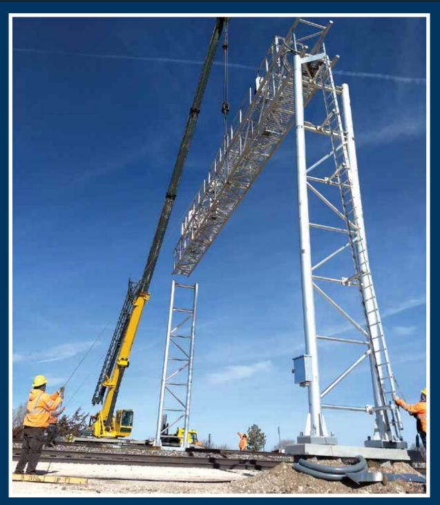
Installation of new bridge signal for siding extension on the Pratt Subdivision MP542.41 (new East Dalhart CPTC542).
