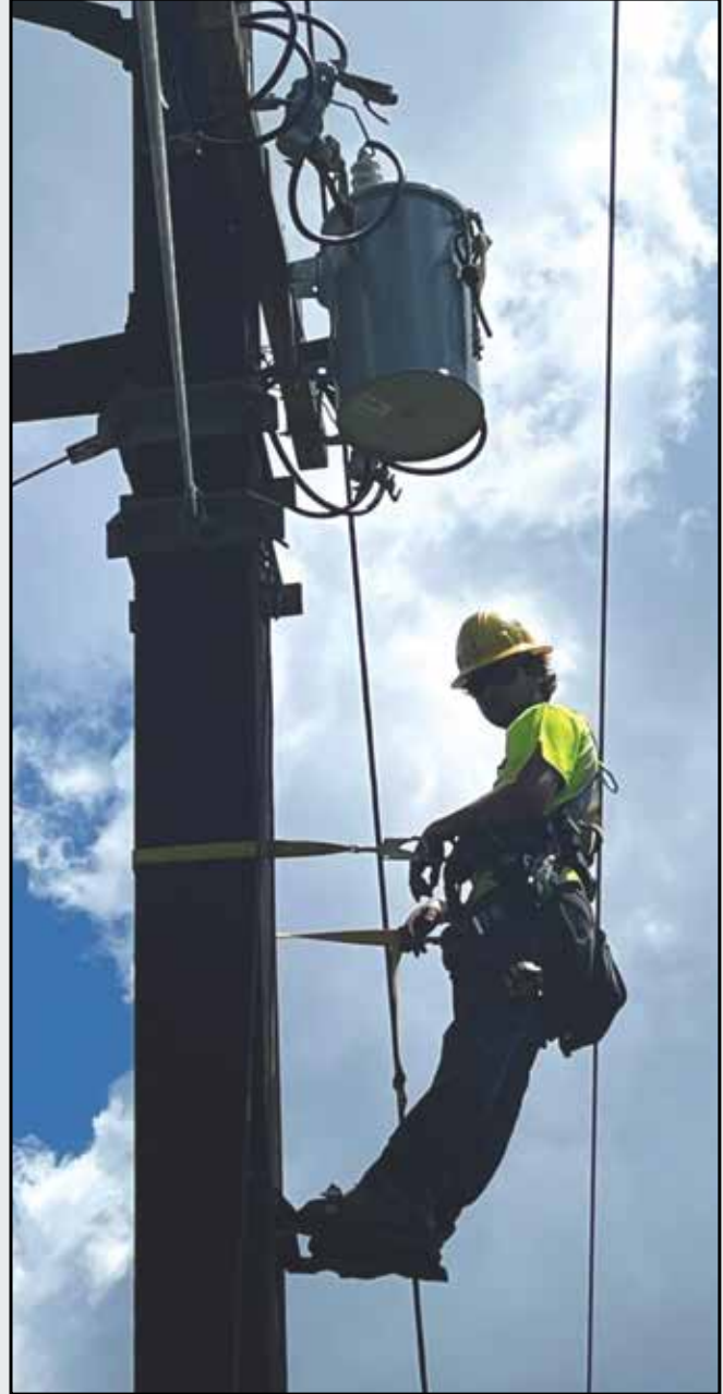
Decklyn Dailey, a Local 53 Signalman Trainee pulls a power cable to a transformer at the Southeastern Pennsylvania Transportation Authority's Breyers Interlocking, West Chester Branch, in Philadelphia, Pennsylvania.
